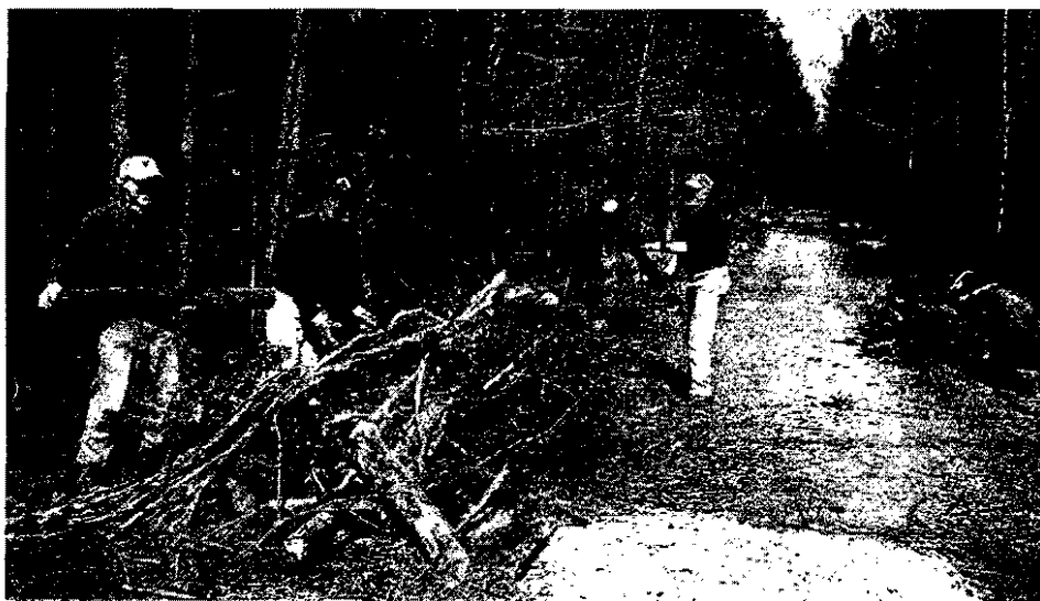
PITCHING IN - TRTC Pres. Bill Bussey, left, gets help from Chris David and Cotten Tyler clearing downed trees from South Durham County section of ATT. Volunteers also are gathering and hauling off truckloads of illegally dumped household trash and construction waste.
